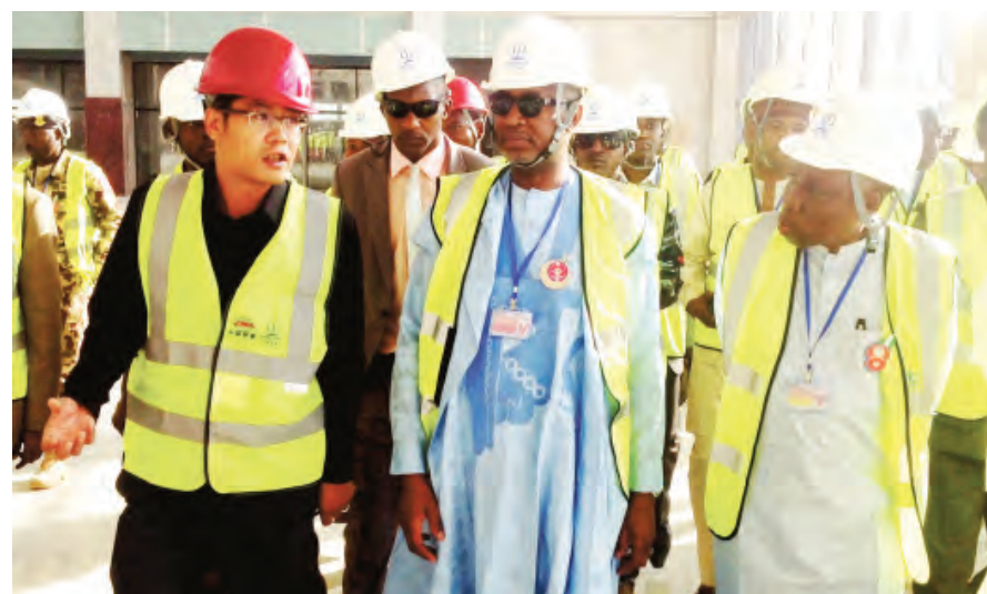
From left: CCECC project manager Mr. Weng Wang, the Minister of State Aviation, Hadi Sirika and the Managing Director, FAAN, Salleh Dunoma at the inspection of the new terminal building under construction at the Malam Aminu International Airport Kano yesterday.
